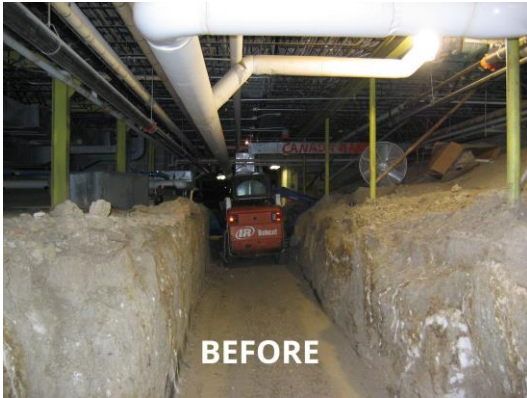
SOUTHEAST HIGH SCHOOL CONVERSION FROM CRAWL SPACE TO BASEMENT, BEFORE AND AFTER TRANSITION
